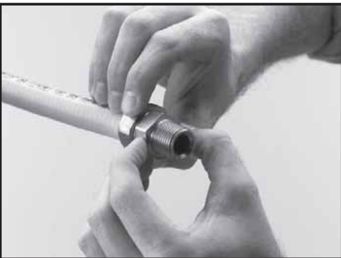
Step 3 Slide nut over retainer and hand-tighten nut to body.
