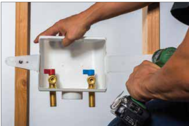
Installation Difficulty. Flimsy box and brackets require extra work and leveling to install correctly.
