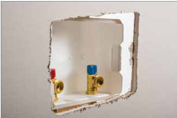
Brackets Are Easily Cut. Rotozip drywall cutters often cut right through thin styrene brackets leaving the plumbing as the only support.
