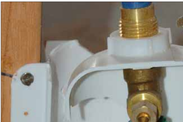
Cheap Materials. Brittle and thin styrene boxes are easily damaged by job site abuse.
