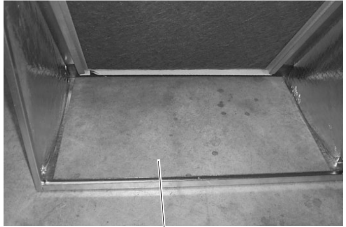
BOTTOM BLOCK OFF PLATE REMOVED
