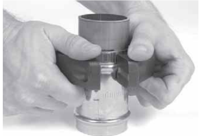
Figure 8 – Installing Press Ring Onto Fitting
