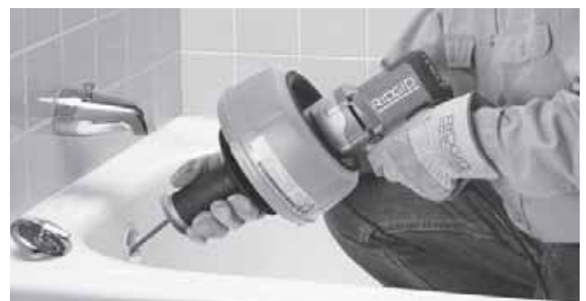
Figure 9 – Push Cable Down Drain Line
