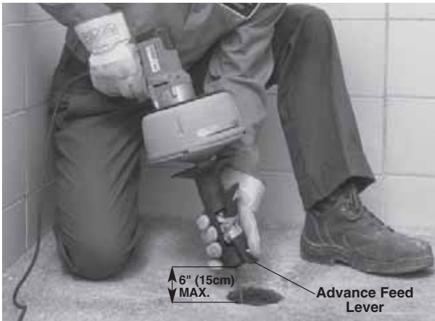
Figure 10 – Feeding Cable With AUTOFEED
