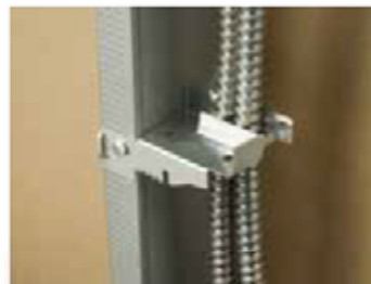
Metal Stud with MC/AC Cable
