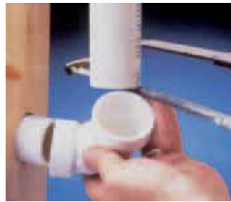
Damaged or leaking fitting is cut out
