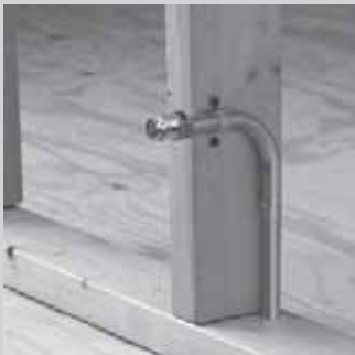
Copper Sweat Stub-Out w/Brass Cap Application
