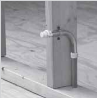
Cold Expansion PEX Stub-Out w/Disposable Cap Application
