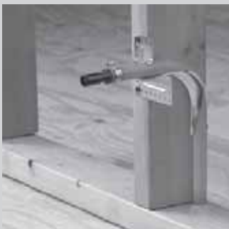
Crimp PEX Application w/Engineered Plastic Stub-Out
