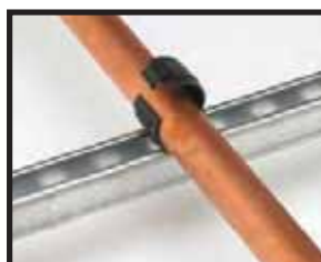
Lay tubing/pipe into clip.
